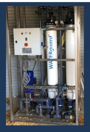
Stand alone water purification system for piped water improvements, rainwater and clean surface water. 100 % guaranteed barrier against legionella, bacteria, micro organisms and viruses.
